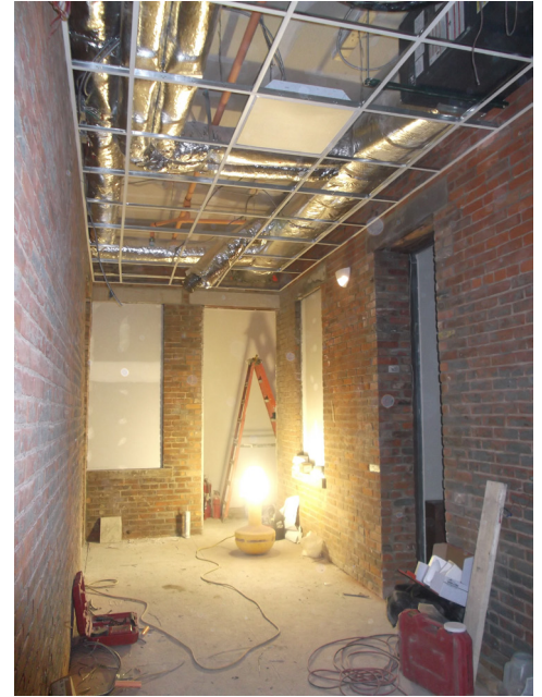
Unfinished interior of an ESSH apartment
