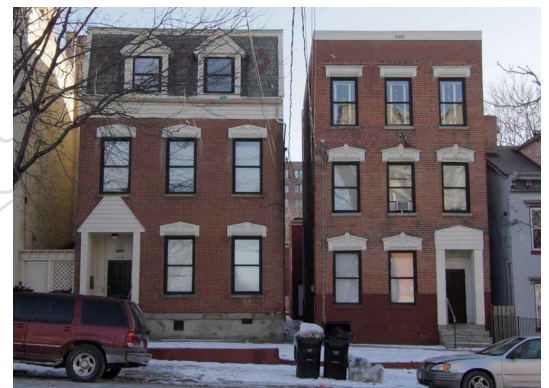
Two of the eight Cutter Apartment buildings
