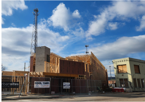
Vandalia Point under construction
